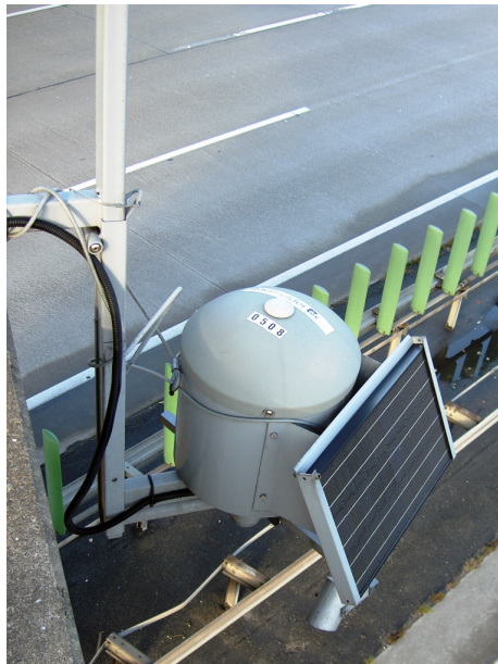
Figure 1.4 – Traffic jam detector in Germany 1 .
